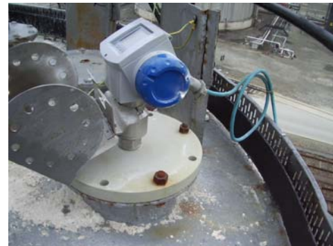
OPTIFLEX for lime level measurement in a silo
