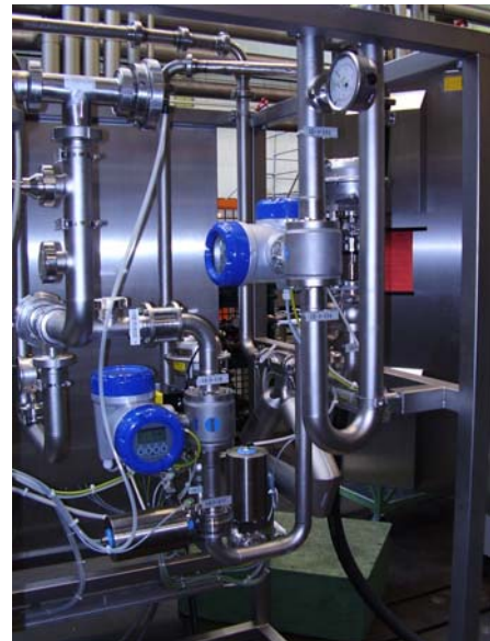
KROHNE's OPTIFLUX is being used to standardise milk to the required fat concentration.
